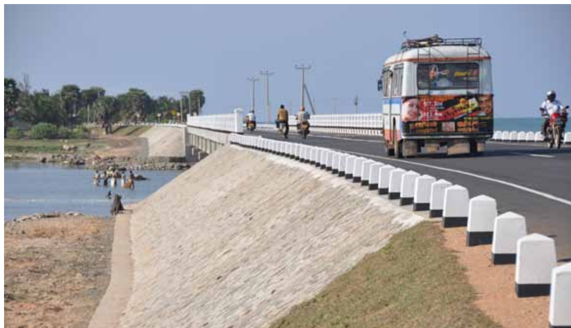
One of two bridges built on Sri Lanka's east coast under the ADB-funded Tsunami-Affected Areas Rehabilitation Project
