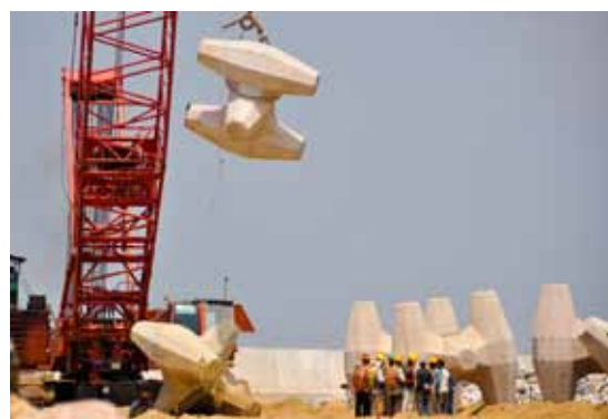
The Colombo Port Expansion Project employs more than 10,000 workers
