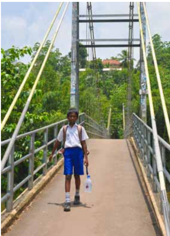
These children no longer risk a dangerous boat ride across a flooded river, thanks to a suspension bridge built under the ADB project
