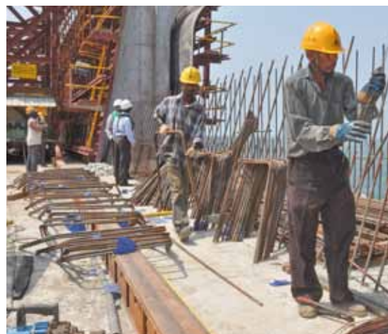
Workers construct the breakwater for the Colombo Port Expansion Project
